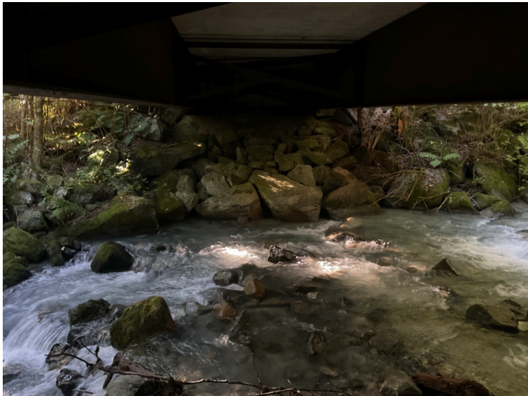
Right Bank Abutment when facing downstream
