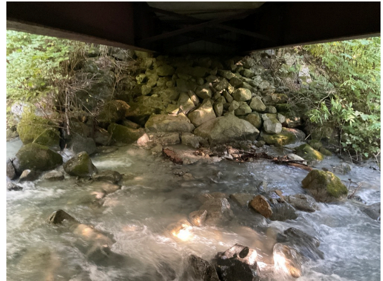
Left Bank Abutment when facing downstream
